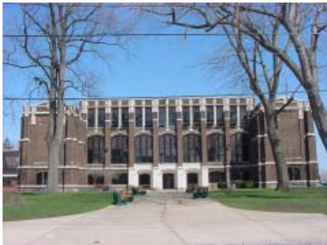
Lakeside High School, Grades 10 through 12
